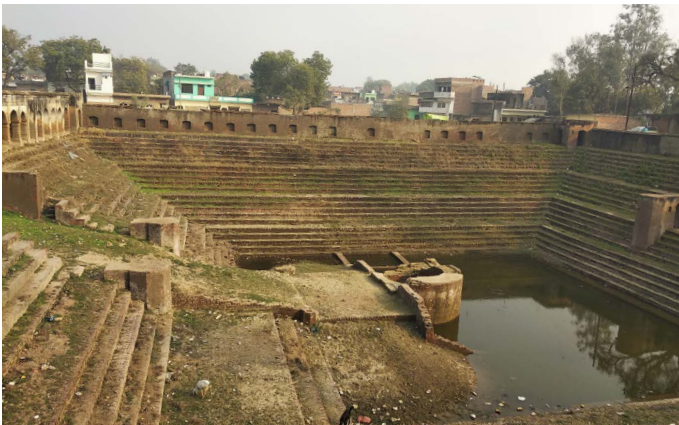
Figure 24 : Pakka Talab, Manikpur Source: Primary survey by AH Division, INTACH Team
