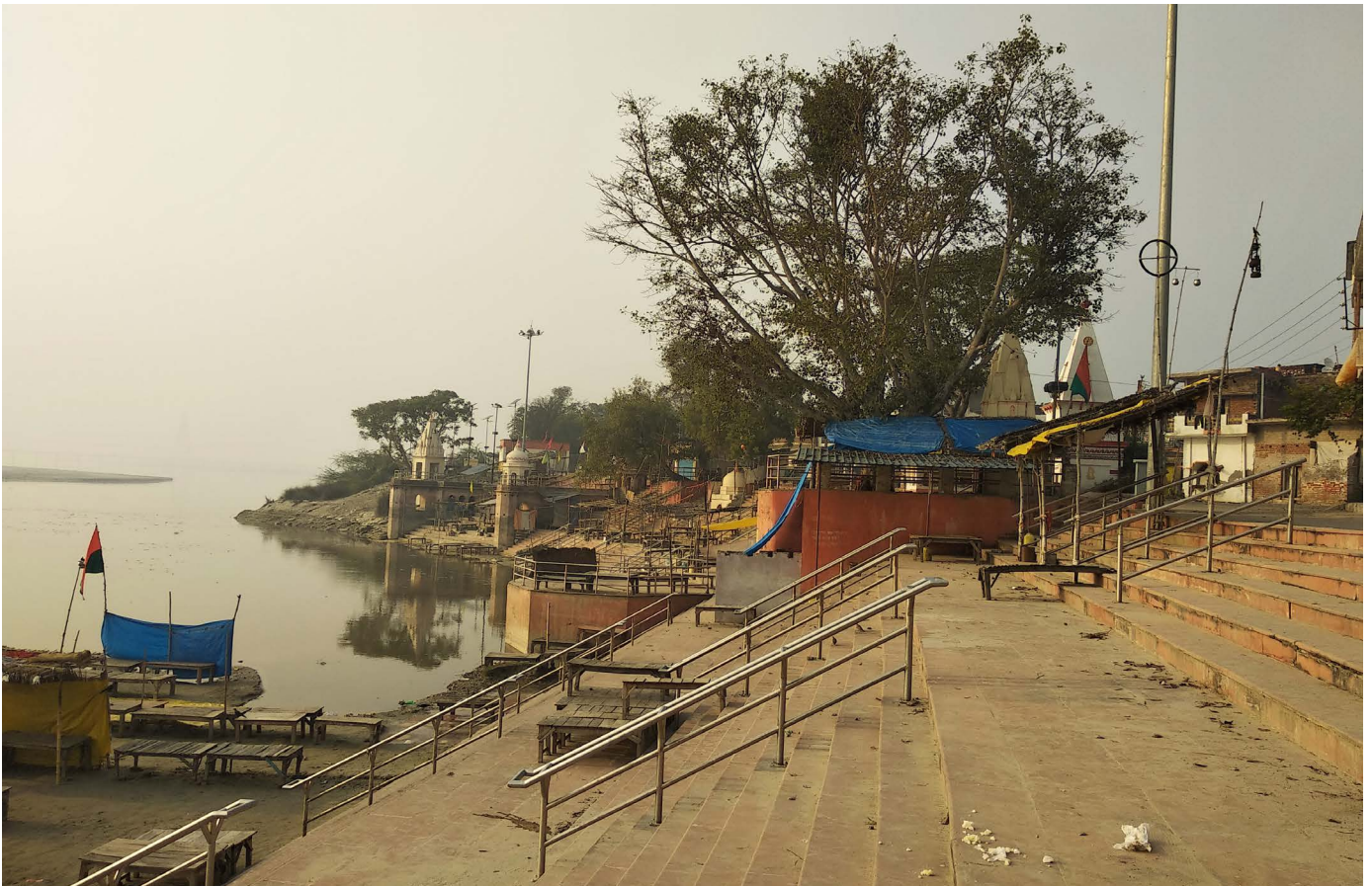
Figure 1 : Ram Janki Ghat, Manikpur. View of ghatscape in Manikpur along river Ganga Source: Primary survey by AH Division, INTACH Team
