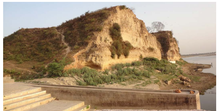
Figure 6 : View of Manik Chand Fort overlooking Ganga, in Manikpur. Source: www.google.com/maps/ , accessed on 16 th June 2022
